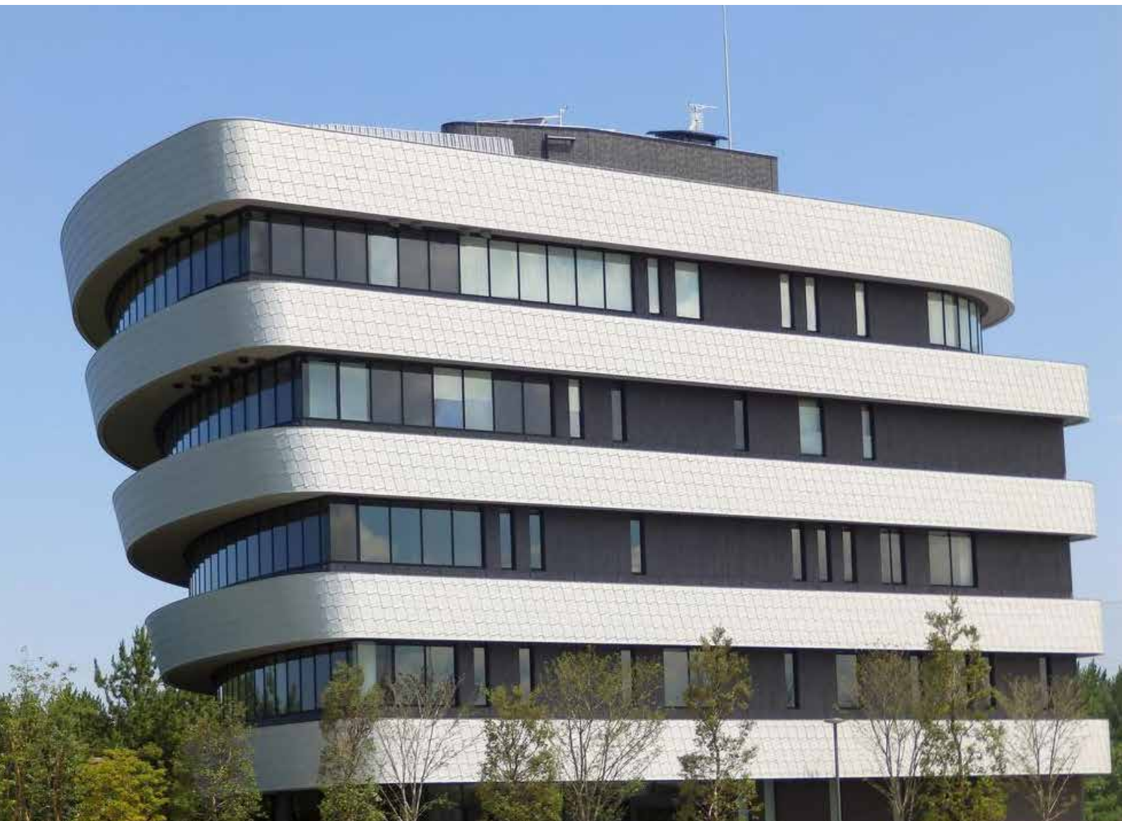
Rinku General Medical Center, Osaka (Japan) - Architect: Nikken Sekkei Ltd. - Technique: VMZINC® Flat lock panel.
